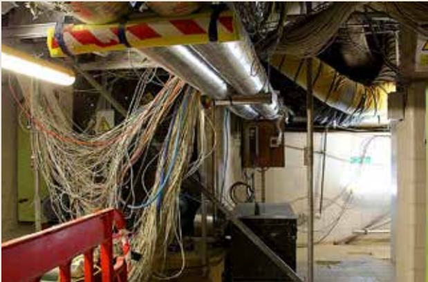
[Top] Fish token found in 2022 [Bottom] Basement cabling
